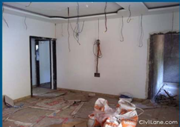
Domestic Electrical Works
