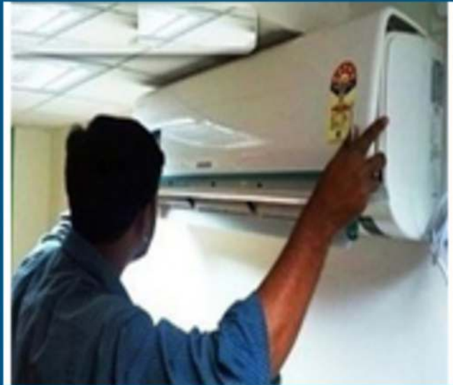
Split AC Intallation
