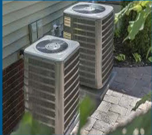
AC Package Unit Installation
